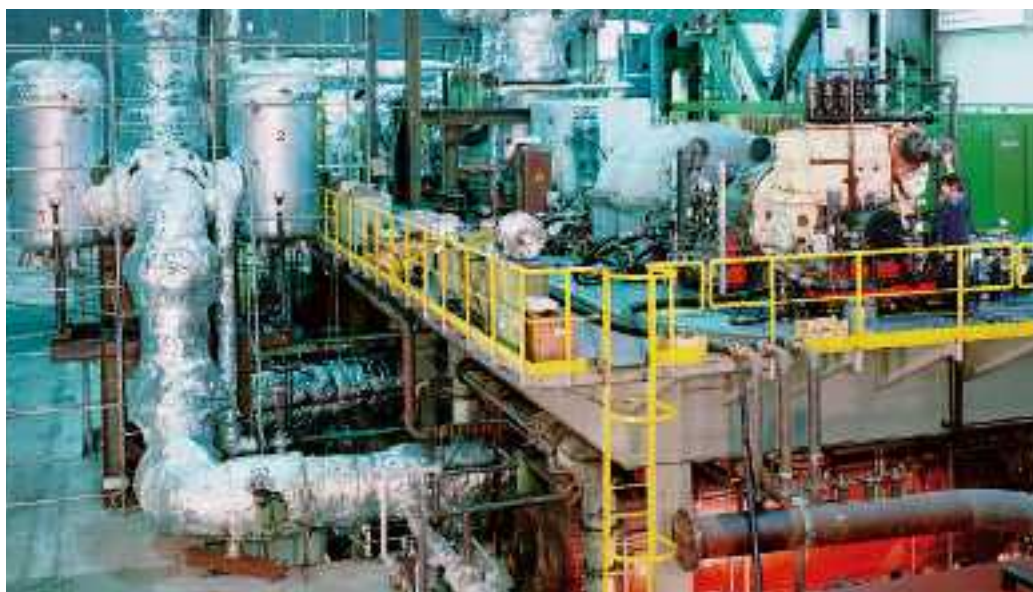
19 Works testing of the machine set for an FCC plant
