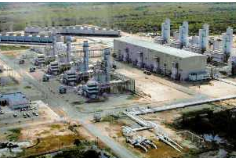
20 World's largest nitrogen production plant
